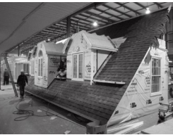
Production of a 28'x40' 4 Box Cape with 3 "A" Dormers
